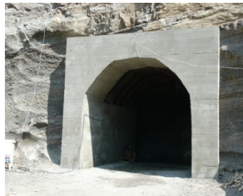
Picture 2. Tunnel adit
