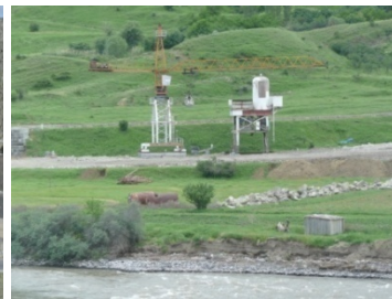
Picture 3. Concrete plant
