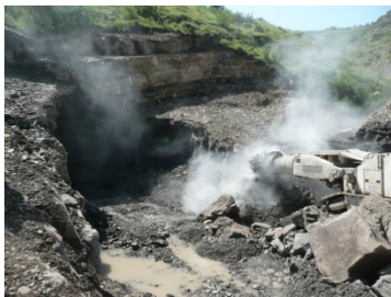
Picture 1. Tunnel adit
