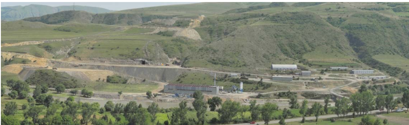
Lower part of the construction site
